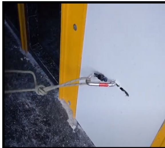
(FIGURE 3, 4) AN ANCHOR AROUND A STUD CAN BE A VERY SECURE ANCHOR, BUT IN THE ABSENCE OF STUDS, A CARABINER ON THE DRYWALL WILL WORK.
